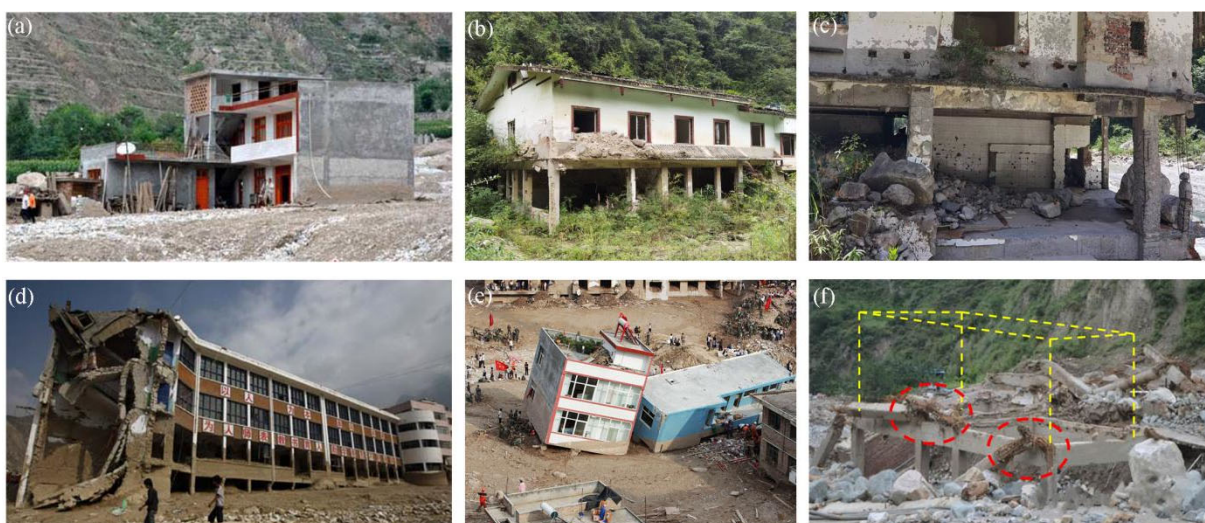
Fig. 1 Building damage scenes in some typical debris flow-affected area. (a) (d) (e) Zhouqu debris flow; (b) (c) Longchi debris flow in Dujiangyan; (f) Qipangou debris flow in Wenchuan. (a) is from www.news.cn ; (b) (c) were taken by the authors; (d) is from business.sohu.com ; (e) is from blog.sina.com.cn ; (f) is from Zeng et al. 2014b).
