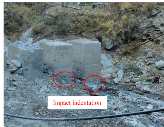
Fig. 10 Impact indentations generated on structures in Li County.
