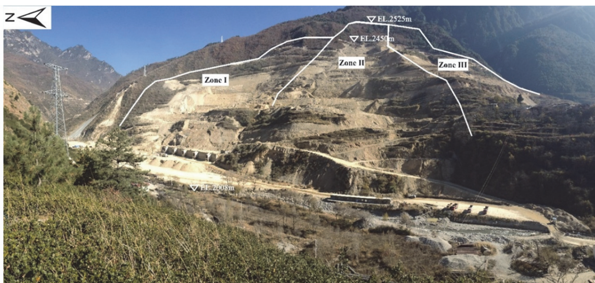
Fig. 1 Slope zoning of the Tangba earth quarry of Changheba Hydropower Station.
