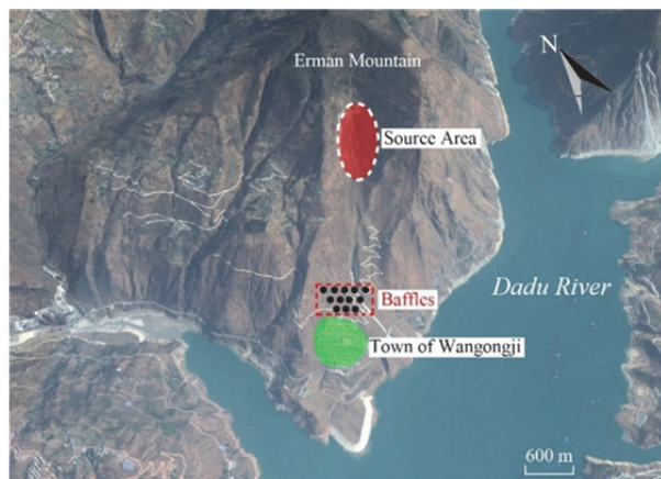
Fig. 1 The geomorphology and engineer layout of Ermanshan landslide (From Google Earth) in Wangongji Town, Hanyuan County, Ya'an City, Sichuan Province.
