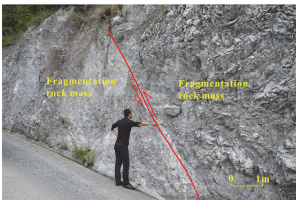
Fig. 4 Fault-induced rock mass fragmentation.
