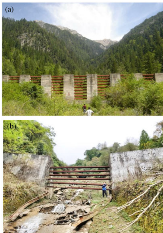
Fig. 1 (a) Typical beam dam in Nuorilang gully, Jiuzhaigou, Northwestern Sichuan, China; (b) Typical beam dam in Lalahu gully, Wenchuan, Northwestern Sichuan, China.
